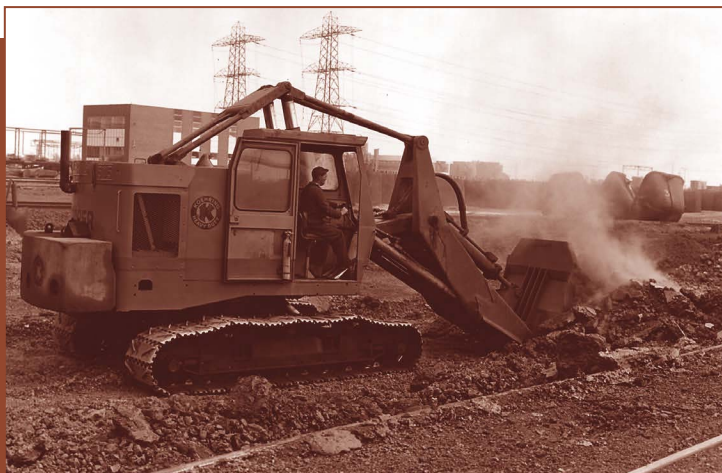
The first Skooper was used on the hybrid Koehring 205 in 1957 and quadrupled the bucket capacity.
